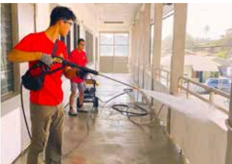
Scout Aaron, along with Scout Leader Chad Fukunaga power washed the second story of the hall on December 14, 2024.
